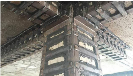
Fig. No. 3.3 Steel jacking in beams and column
