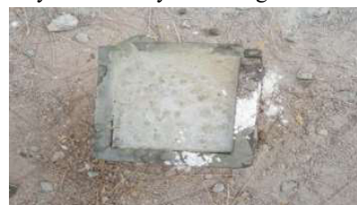
Casting of cubes
